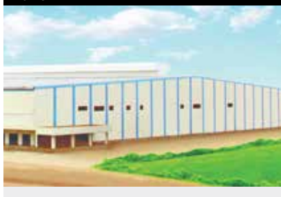
Reliance National Distribution Centre, Pune
