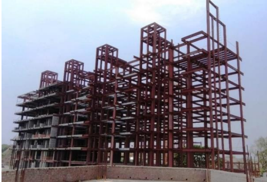
High-rise structure in Hyderabad
